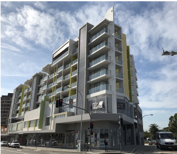
Photograph 13. The 7 storey Hurstville Times Plaza development has frontage to Forest Road, Alfred Street and Treacy Street.
