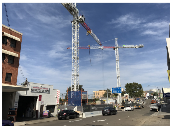
Photograph 16. Currently under construction
