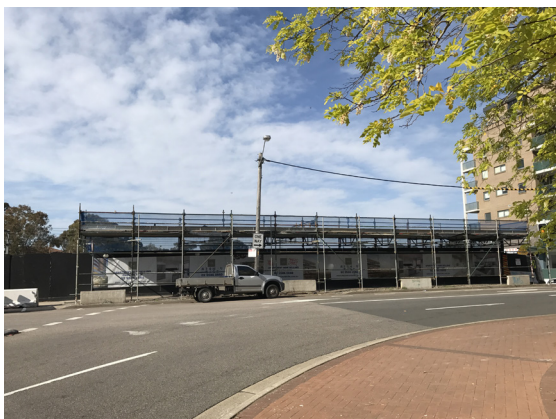
Photograph 9. 1-5 Treacy Street currently under construction to 9 storeys.
