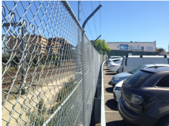
Photograph 2. Chain mesh fencing, block wall retaining and a vehicle barrier separate the subject site from the railway reserve.
