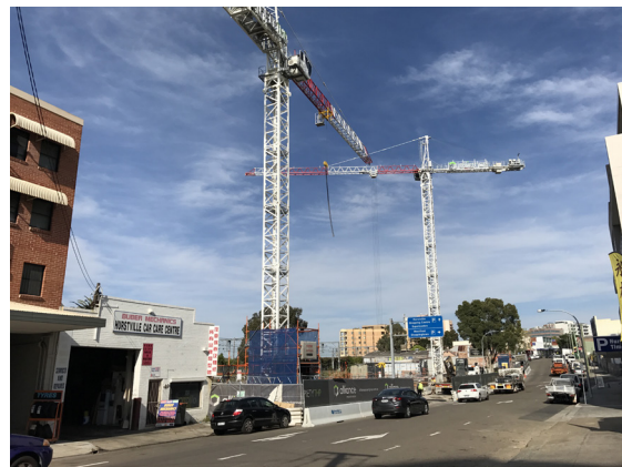
Photograph 8. 21-35 Treacy Street currently under construction
