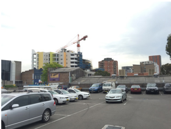
Photograph 3. The eastern boundary is separated from the neighbouring site by chain mesh fencing, block wall retaining and a vehicle barrier.
