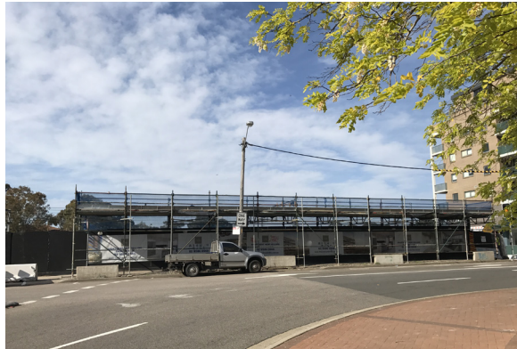
Photograph 19. 1-5 Treacy Street currently under construction
